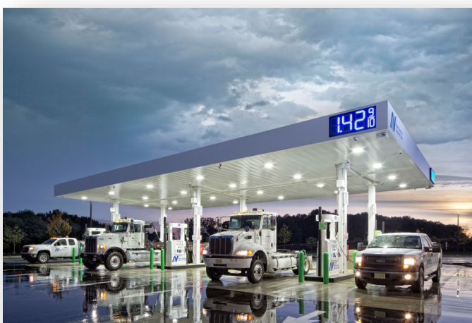
CNG Fueling Station
