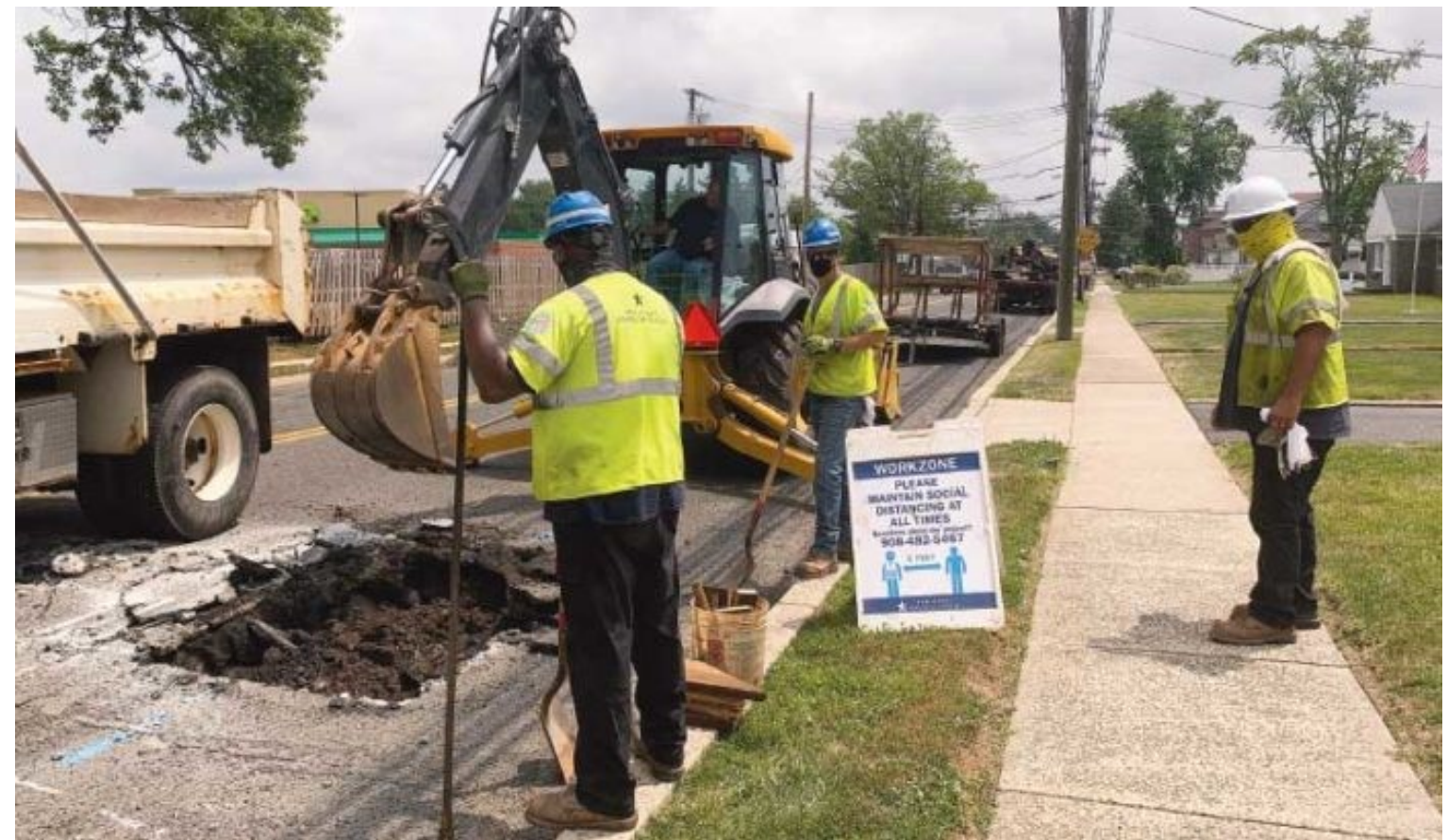
New Jersey American Water workers replacing a fitting while social distancing.
