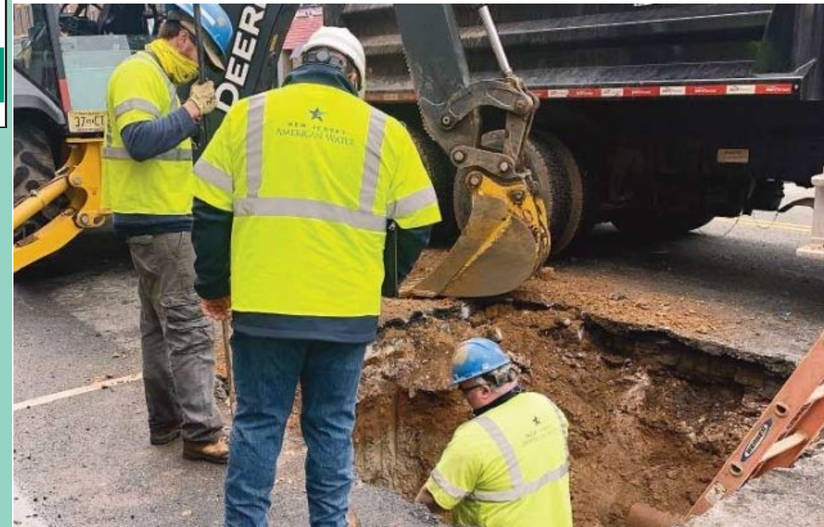
New Jersey American Water workers. fixing a water main break in Westfield. - Photos courtesy New Jersey American Water
